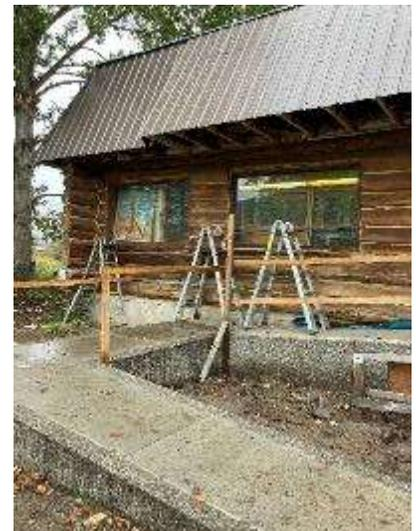
The old shake roof and plywood soffits are being replaced with metal to improve the Nature House and reduce fire risk as part of the overall “Fire Smart” plan for the Nature Centre property. Come and check it out. I think it looks classy and modern but also fits in well with the natural setting.
