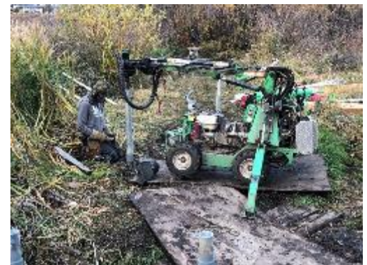
Reece Hoath installing pilings
